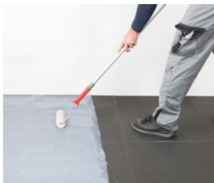
Application of the pressure sensitive adhesive
