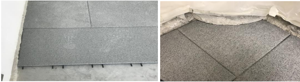
Start the second row shifted by a half tile; cutting of a round corner
