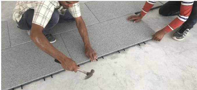
Closing the gaps with a hammer
