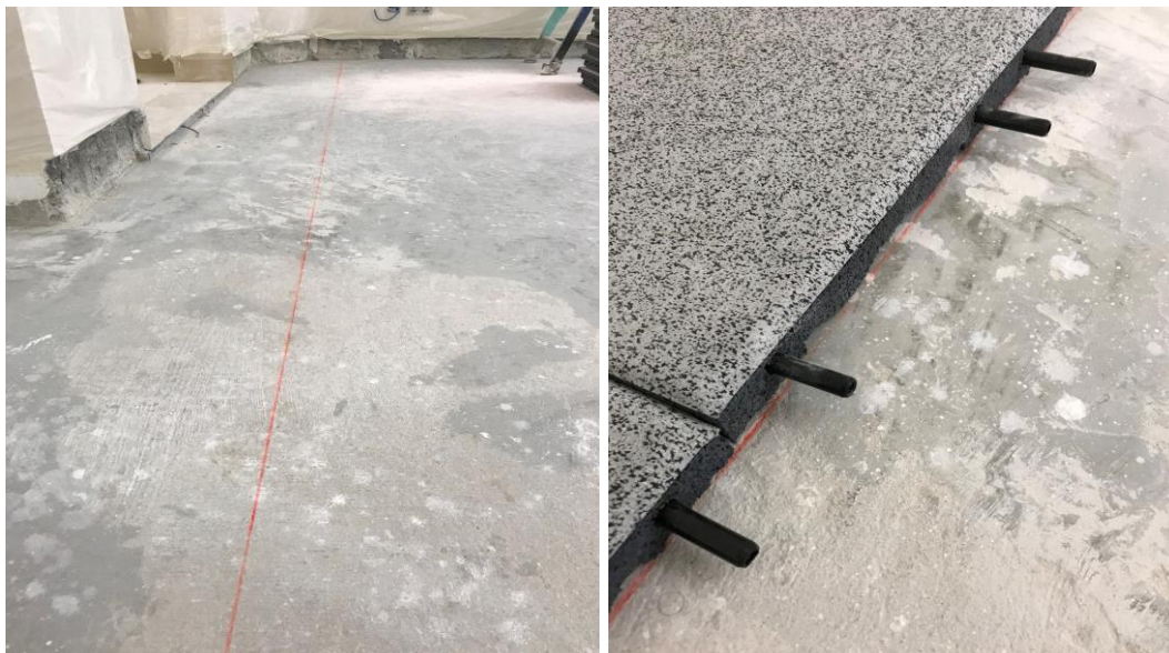
Creating chalk lines and laying the tiles along this line
