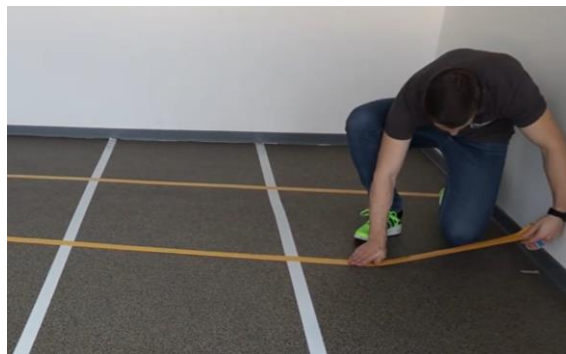
Pull-off foil of adhesive tapes in longitudinal direction, apply adhesive tapes in transvers direction
