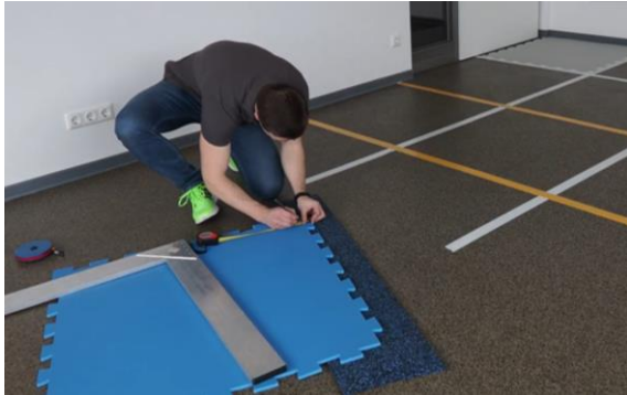
Create a straight edge without teeth and lay the mats along the wall
