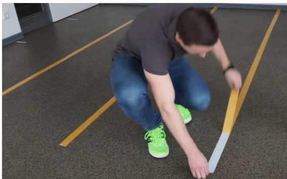
Pull-off foil of adhesive tapes in longitudinal direction, apply adhesive tapes in transvers direction
