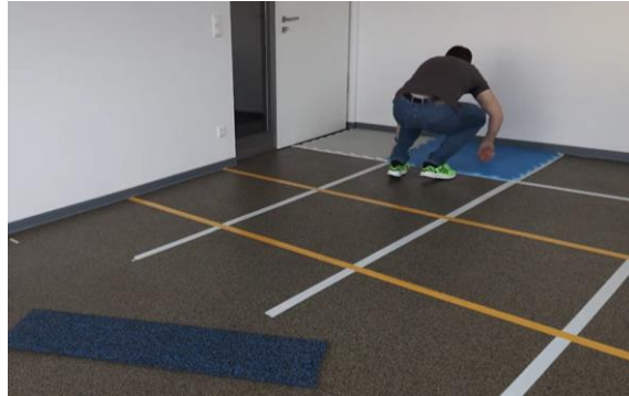
Create a straight edge without teeth and lay the mats along the wall
