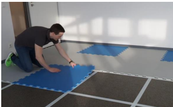
Connect mat by mat and fix it to the floor
