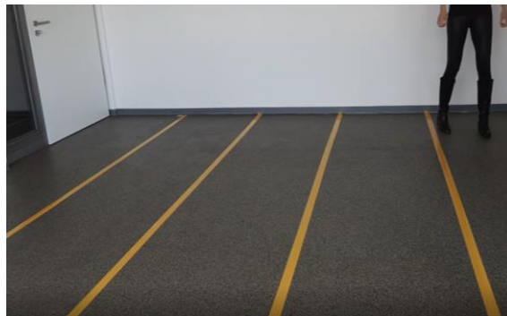
Measuring the lanes for the adhesive strips and application of adhesive tapes in longitudinal direction
