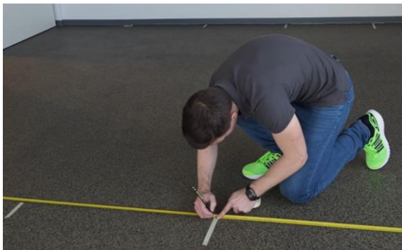
Measuring the lanes for the adhesive strips and application of adhesive tapes in longitudinal direction
